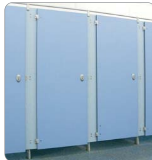
Toilet cubicles at Wreake Valley College
